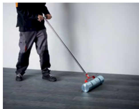
b - Smooth down the entire flooring area using the large, heavy roller.
