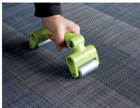
a - Smooth down the joints using the small seam roller.
